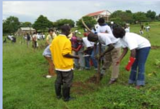
UNVs Akello Carolyn and James Ojok (1st and 2nd right) were part of the team that put up the barbed wire fence to protect the planted seedlings at Entebbe Comprehensive School
